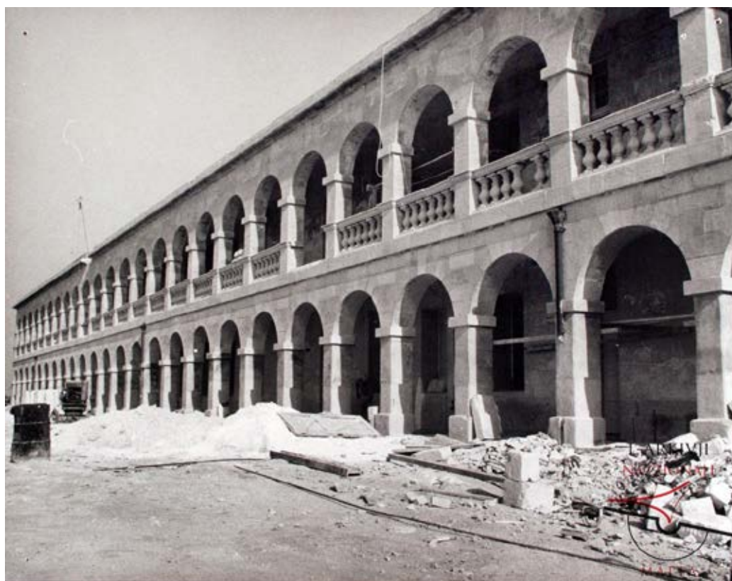
Another view of Barracks during 80s works
