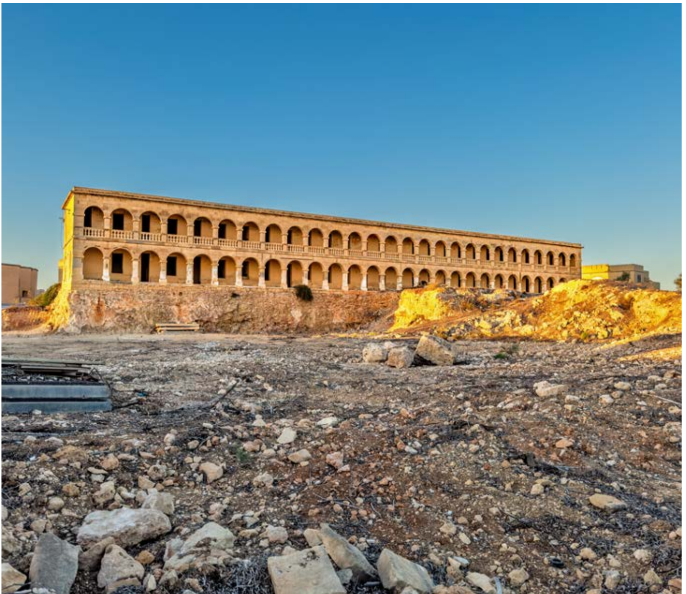
FIG. C: The south facing arcaded façade of the British Married Quarters Late Victorian Barracks in Fort Chambray.
