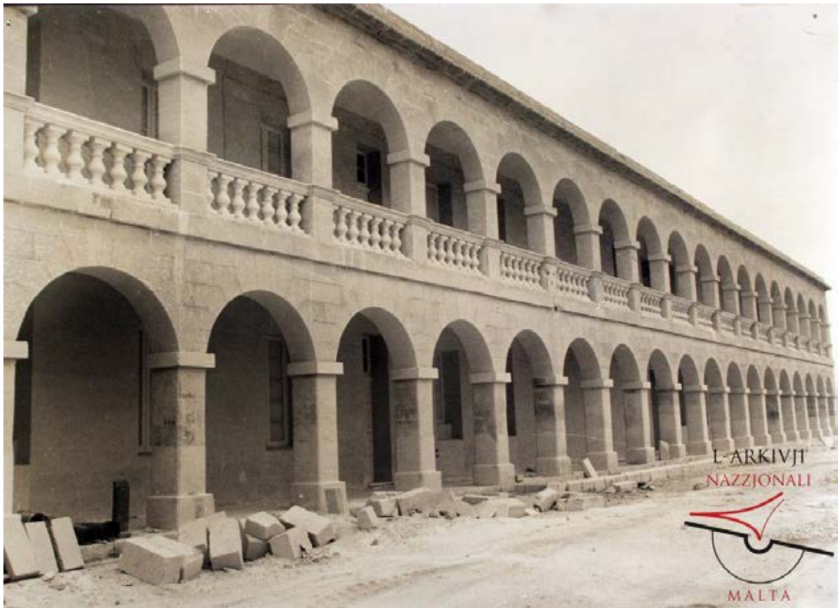
View of Barracks during work being undertaken in the 80s for use as tourist accommodation
