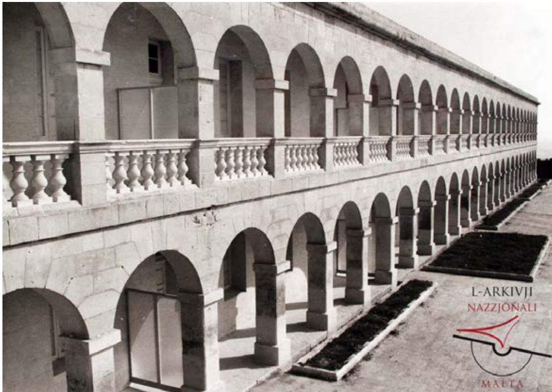
View of Barracks arcades
